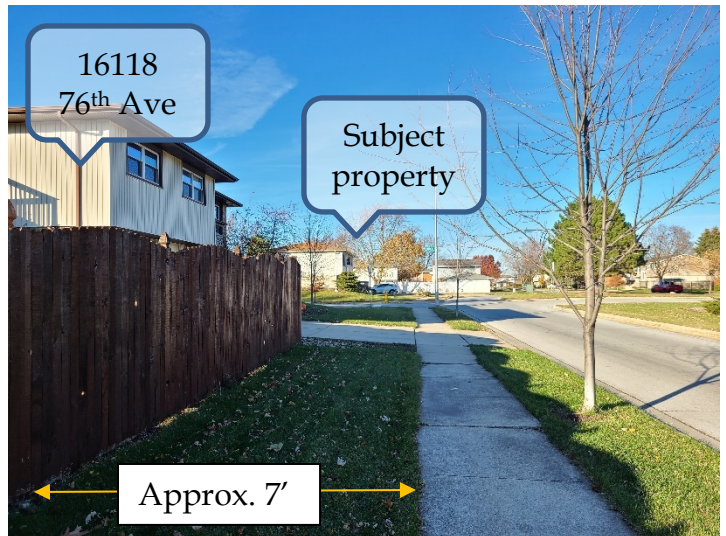
Existing fence approximately 7 feet from west edge of sidewalk at 16118 76th Ave (south of subject property as shown in the background)
